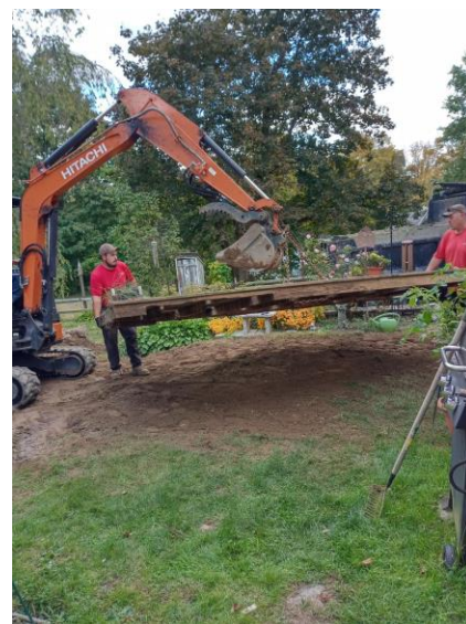
Removing back deck
