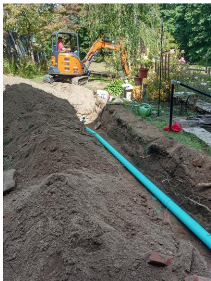
New sewer line
