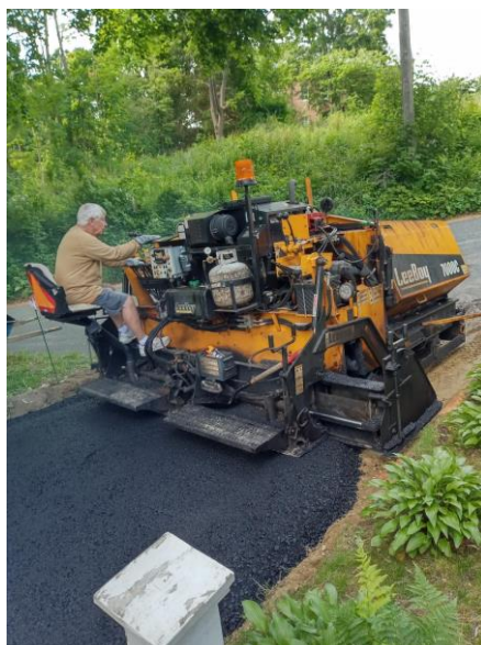
Paving back driveway
