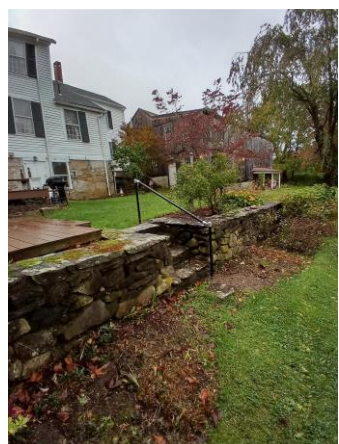
New stair handrails
