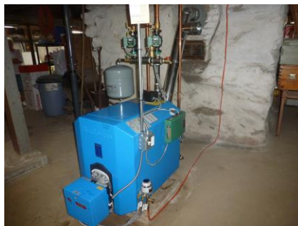
New Tavern furnace
