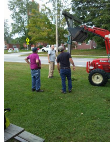
Work crew of Bob Ducharme, Dave Proulx and Will Moseley erect repaired post.
