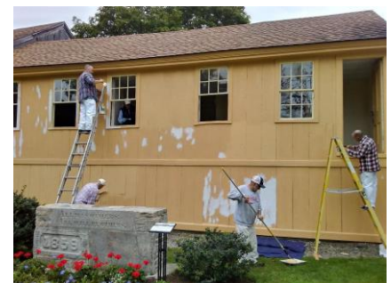
Work crew consisting of Bob Grzyb, Ken Butkiewicz, Ed Bazinet, Bob Ducharme and Tim Cushing painting the annex.
