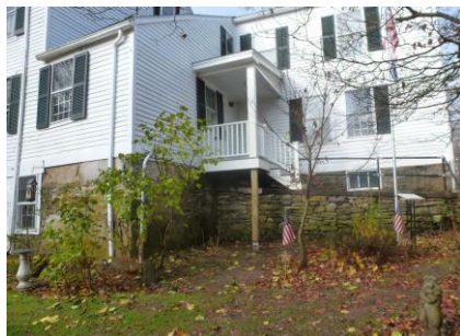
New upgrade to the rear entrance/exit of the Tavern.
