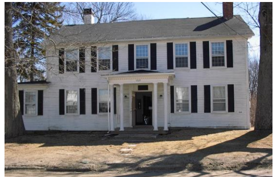
1805 House prior to its demolition
