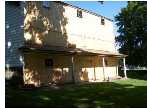
Completed east wall of barn
