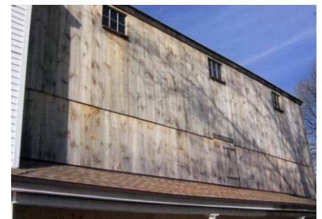
Back of Barn Renovations
