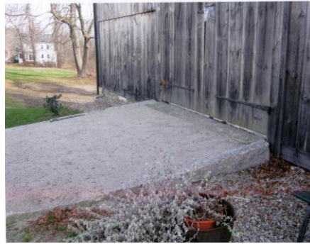
Handicap Ramp at Front of Barn
