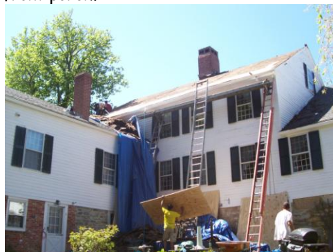
Rudnicki Roofing replaces the Tavern roof.
